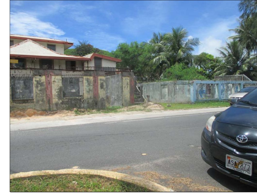
Current View showing Elevated Roadway Improvements & Elevated Sidewalk
