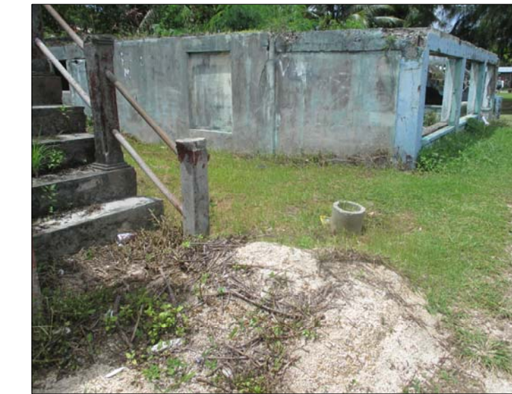
Exposed Concrete Slab buried under Elevated Grade at adjacent Meno House (Chargulaf house in the background)
