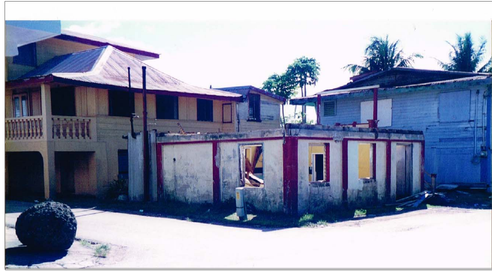
Side Elevation Charqualaf House (right side of photograph)
